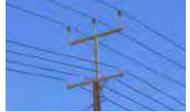
High voltage and low voltage on same pole
