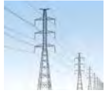
High voltage transmission
